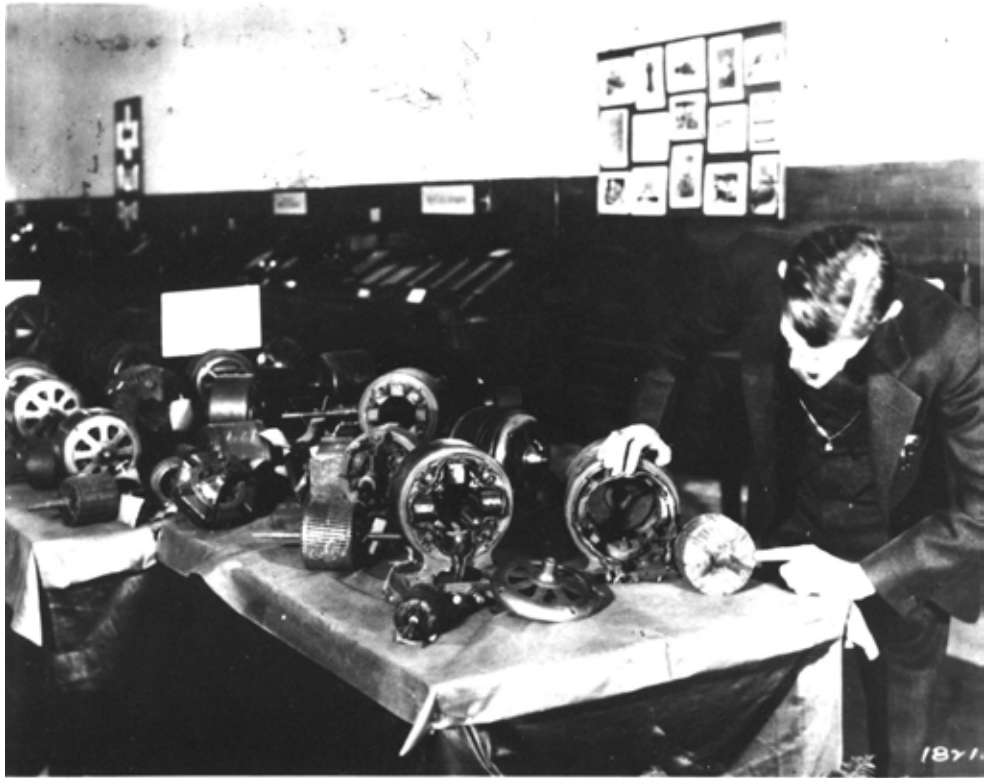
Nikola Tesla Introduces His Revolutionary Polyphase A.C. Induction Motors At The Columbian Exposition
